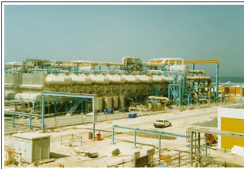
Figure 11. Multi Stage Flash Desalination Plant at Jebel Ali G Station, UAE.
